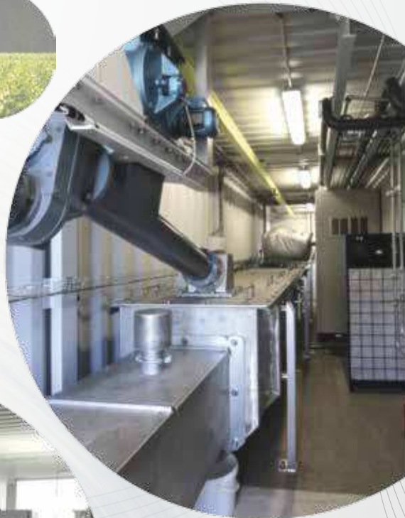
Inside the full containerized plant for 10 000 PE
